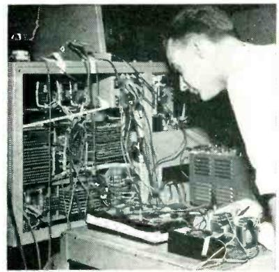
Magnetic amplifier test setup, showing use of masking tape for anchoring additional selenium rectifier on top of cabinet and for supporting glass thermometer
