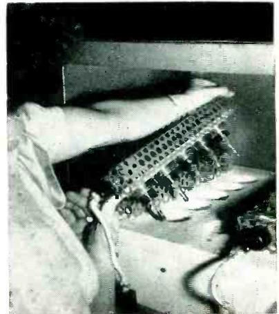
Rack for holding five subminiature tubes at a time inside high-temperature oven.
