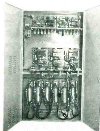
Front view of welder control unit, with doors open
