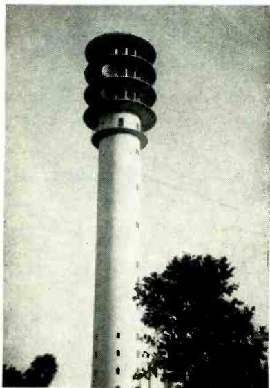
Microwave relay links new German tv stations. Tower houses repeater station
