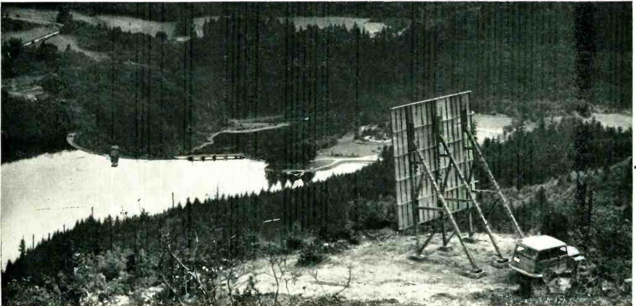
Signal path from the passive repeater (right, compared with jeep) lies over Merwin Dam to the station just visible (upper left)
