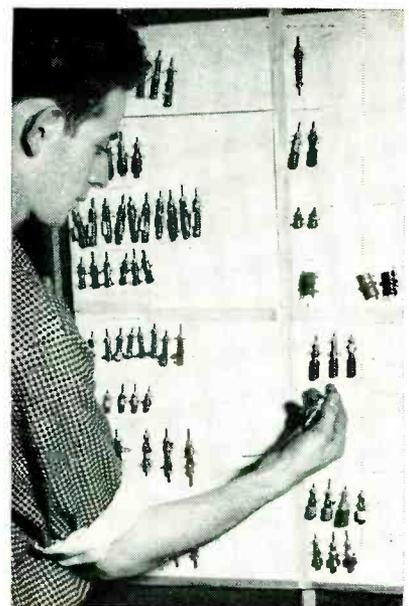
Using coil sample board to identify a defective unit. Vendors are identified on board by code letters, generally the first letter in the company name. Loops of wire pass through holes in board to hold each sample in position
