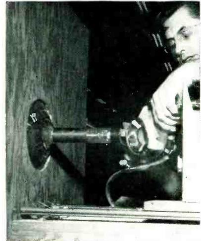
Placing 90-degree yoke over neck of 30-inch picture tube in DuMont test set
