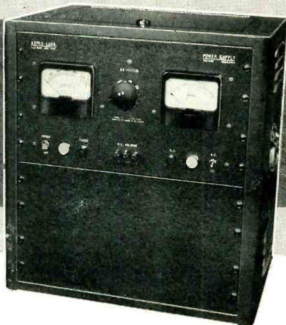
The Kepco Model 700 features one regulated voltage supply with excellent regulation, low ripple content and low output impedance.
