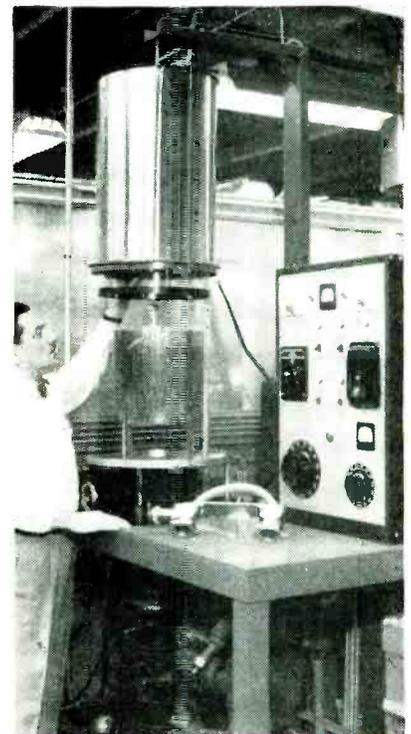
Bakeout equipment with bell jar and oven lifted to show basket in which parts are placed for final degasification. Large part on bench is an analyzer tube for a mass spectrometer, one of the largest parts customarily baked out
