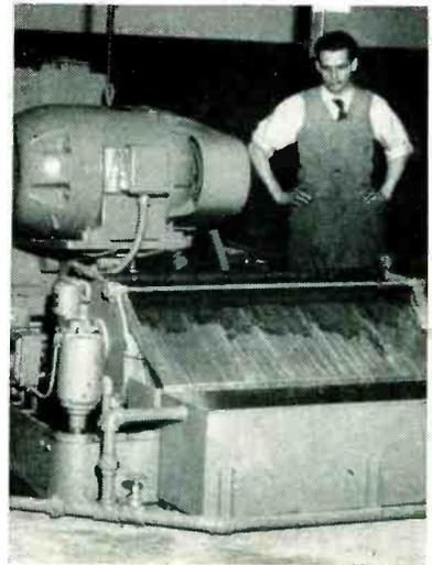
Alnico particles slide down metal incline to bin in foreground after being scraped off drum of magnetic separator, here installed on Besly No. 226 double-end grinder
